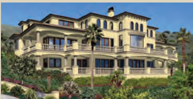
10 Bluff Drive, Shell Beach New Construction - Completion: Fall 2008
